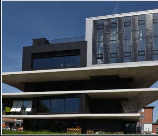
roof & facade installation
