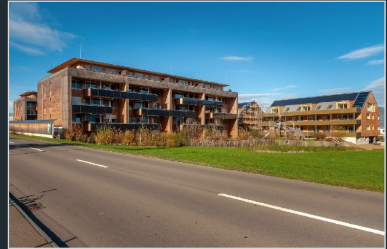
roofs and balconies
